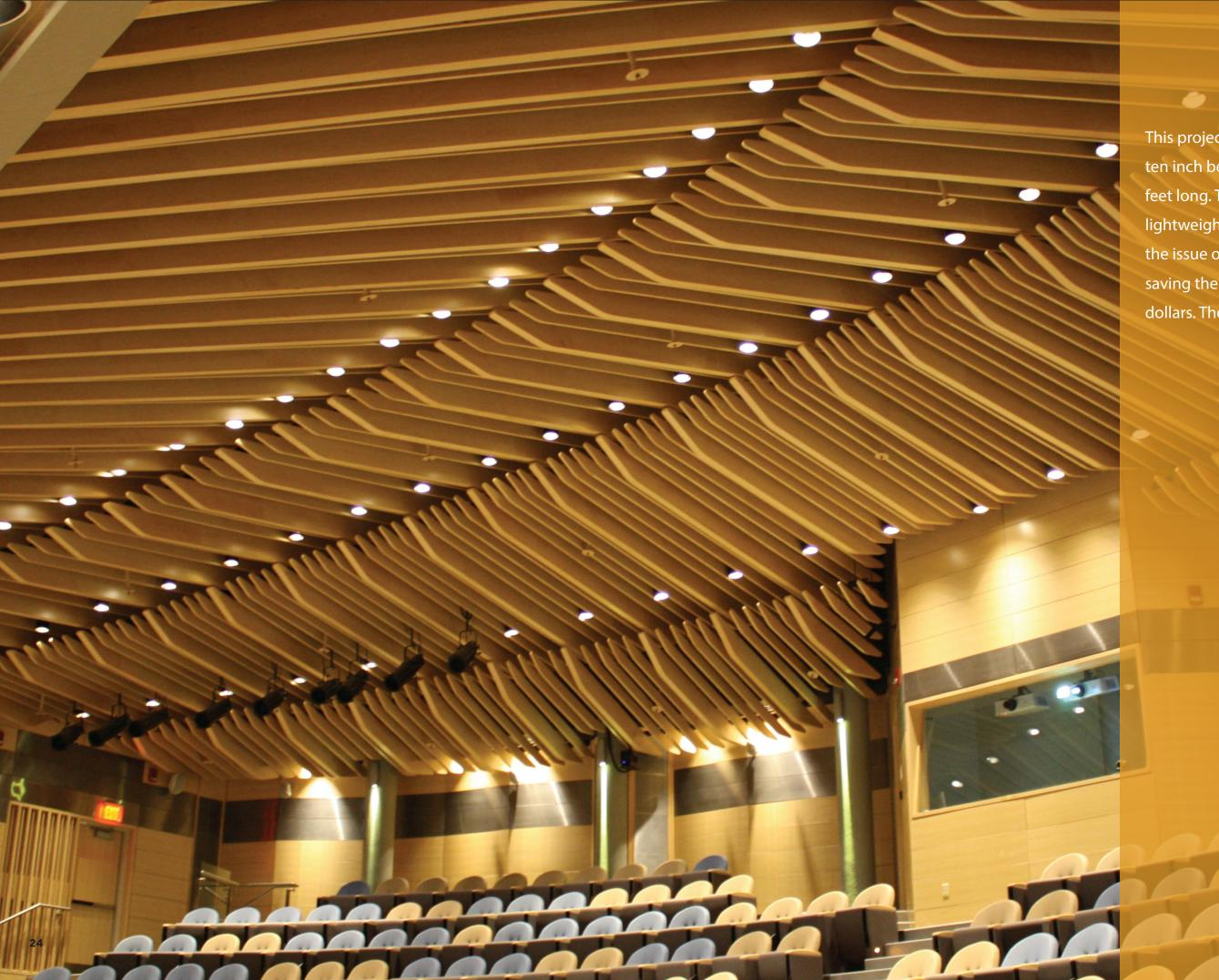
This project required three inch by ten inch beams up to twenty-seven feet long. This was achieved using lightweight technology, solving the issue of support structure and saving the client thousands of dollars. The result is spectacular.
